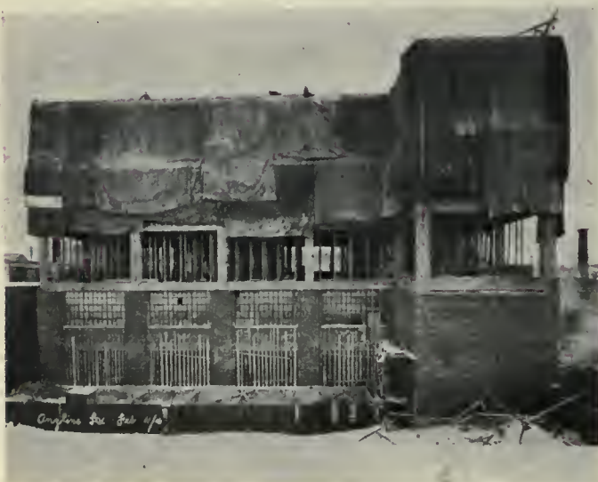
Buildings closed in with tarpaulins—Feb. 11, 1916.
